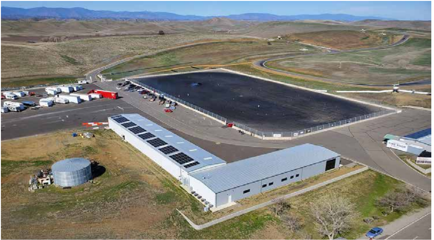
Skid pad and additional shop space.
