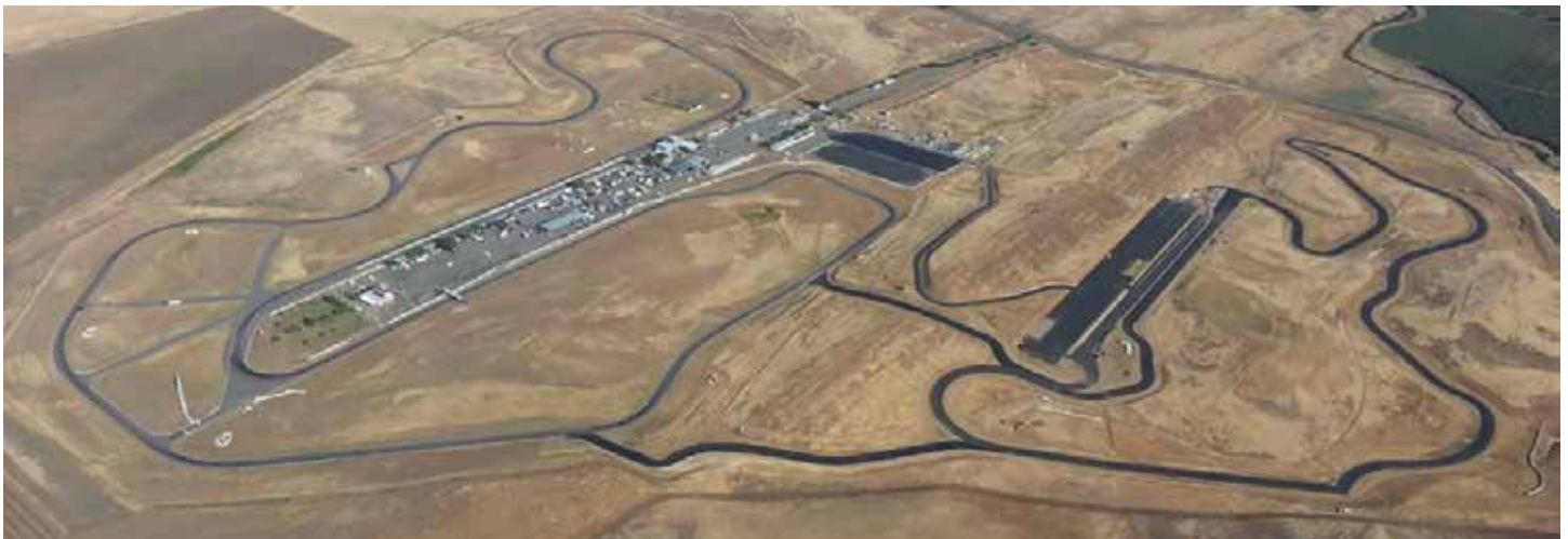
Aerial view after West Course was completed.
