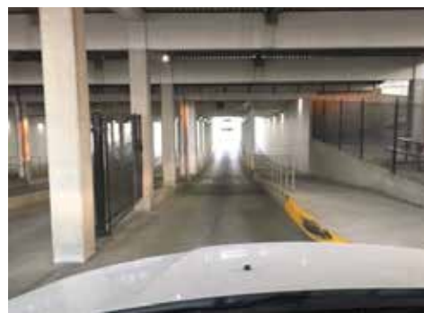
The tunnel under the track leading into the infield
