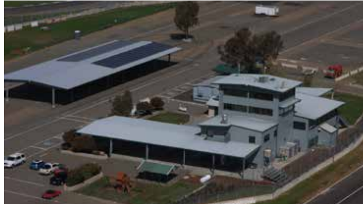
Thunderhill continues to embrace green with over 325 solar panels located on the tops of just about everything. The solar effort offsets approximately 70% of the annual Thunderhill P. G. & E. service costs.
