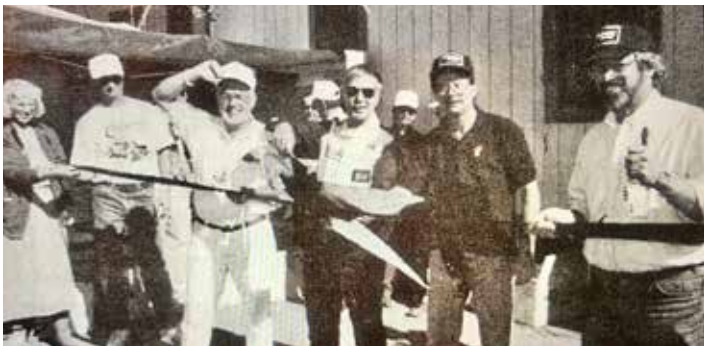
TRP groundbreaking Oct 1993
