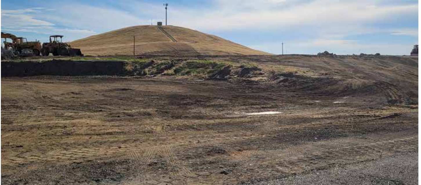
Progress on hill removal
