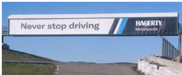
Newly completed Hagerty bridge
