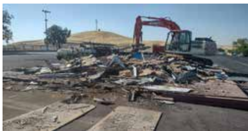
Destruction of the old store in progress
